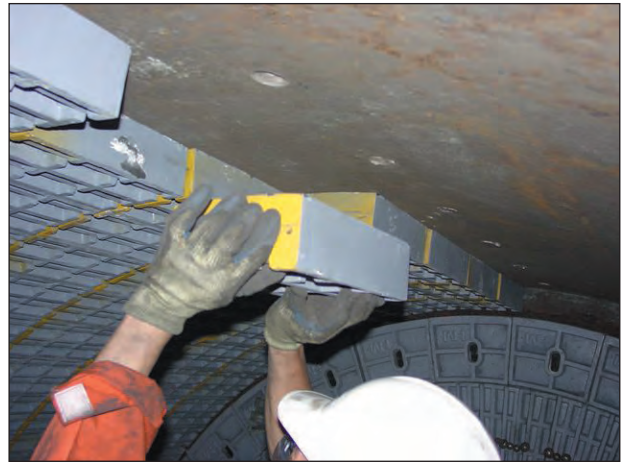
A magnet holds the liner to the mill shell.
